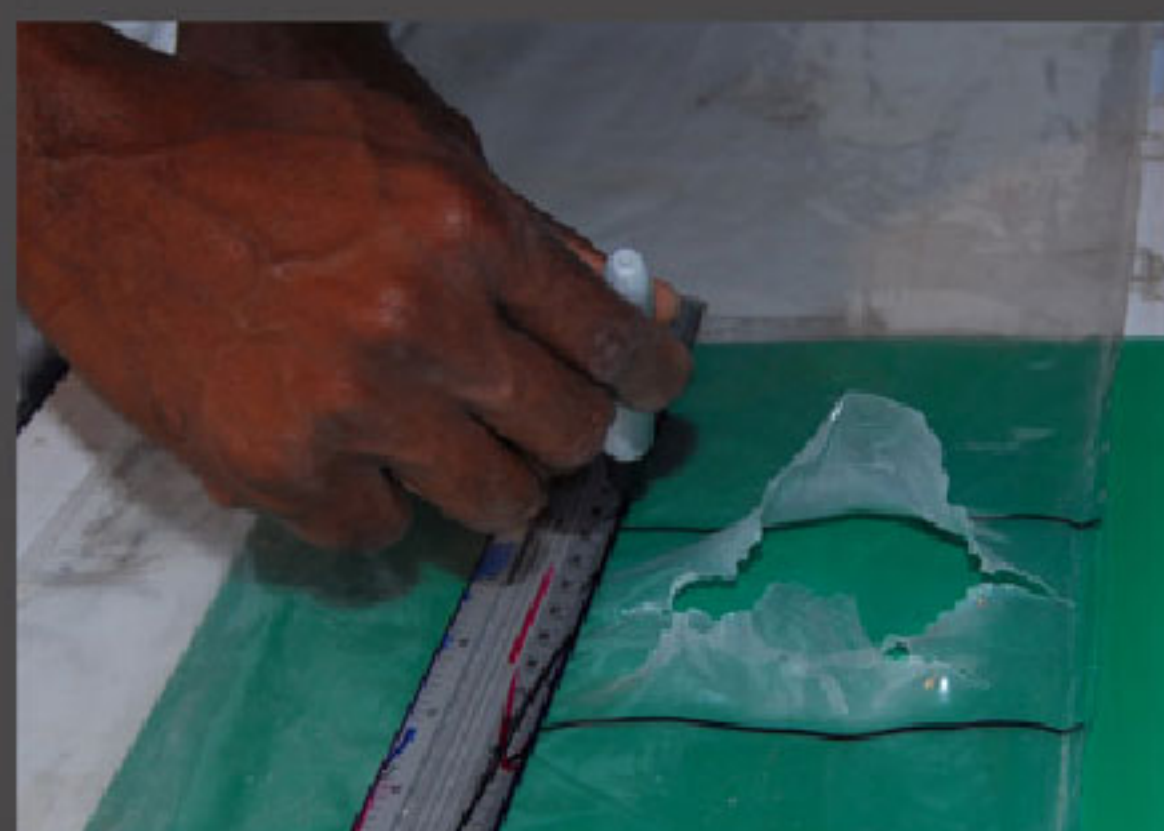
Secure the bladder with masking tape so that it will not move while you work. Clearly mark your work area with guide lines and cut all damaged and stretched materials away
